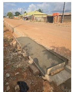
Stormwater culvert
