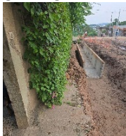
Deep drain 3 feet from our gate entry
