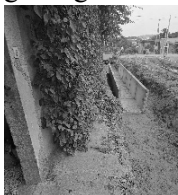
Deep drain 3 feet from our gate entry
